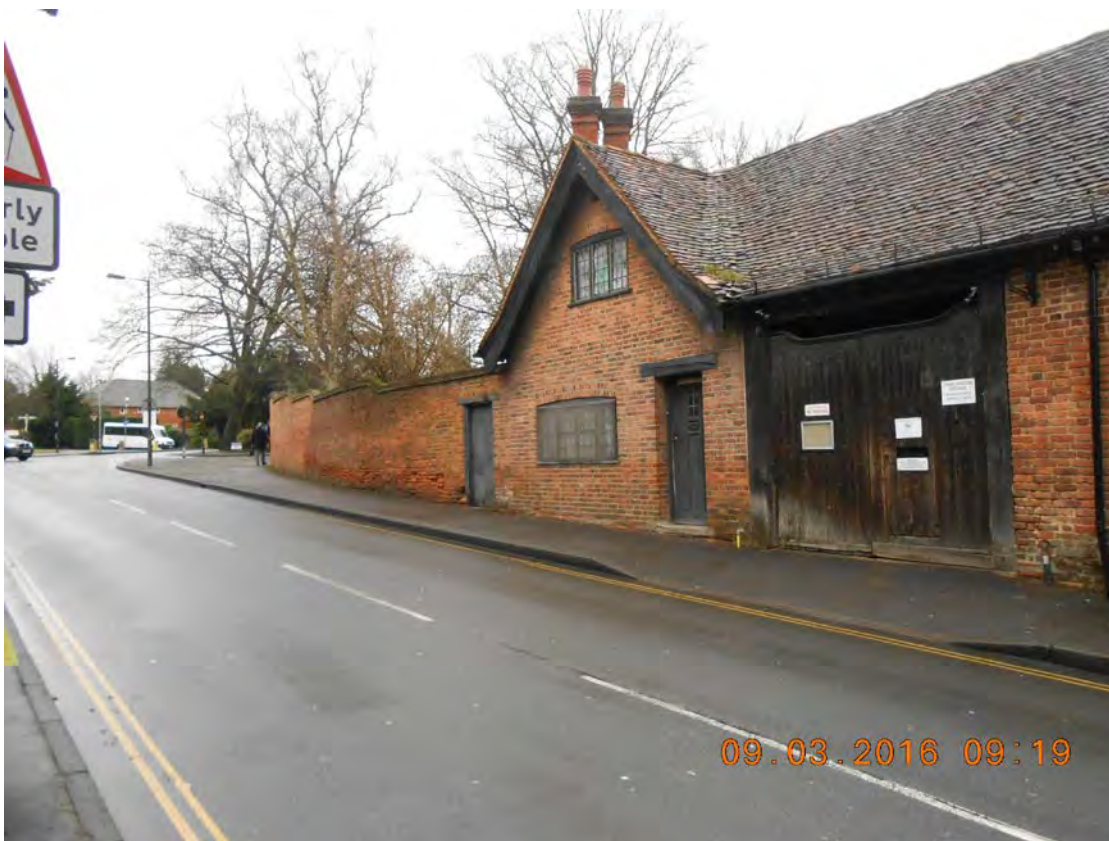
EXISTING COTTAGE FROM OLD CHURCH LANE
